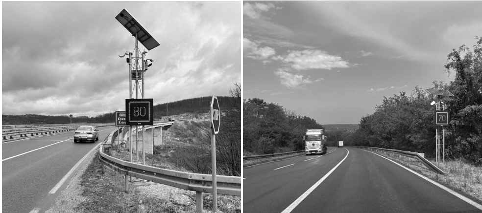
Figure 1. Smart Traffic Sign for Advisory Speed
